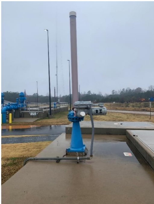
Photo 2 - 108" Slide Gate Actuator at Junction Box Structure
