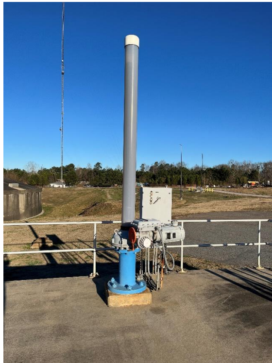
Photo 5 – 108” Slide Gate Actuator at Overflow Structure
