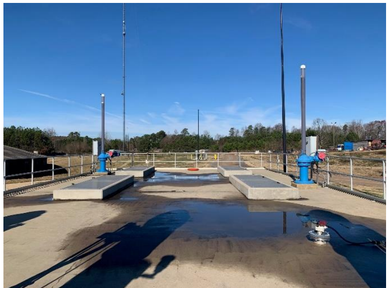
Photo 3 - 108" Slide Gate Actuators at Flow Diversion Structure
